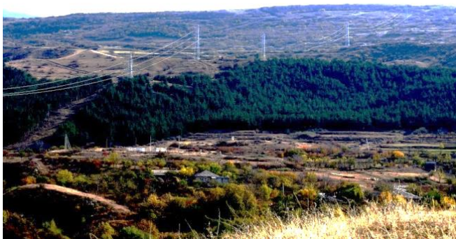
Figure 5. ETL section at Damala village.
