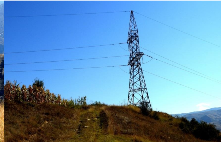
Figure 5. Section of ridge crest near № 99 tower.
